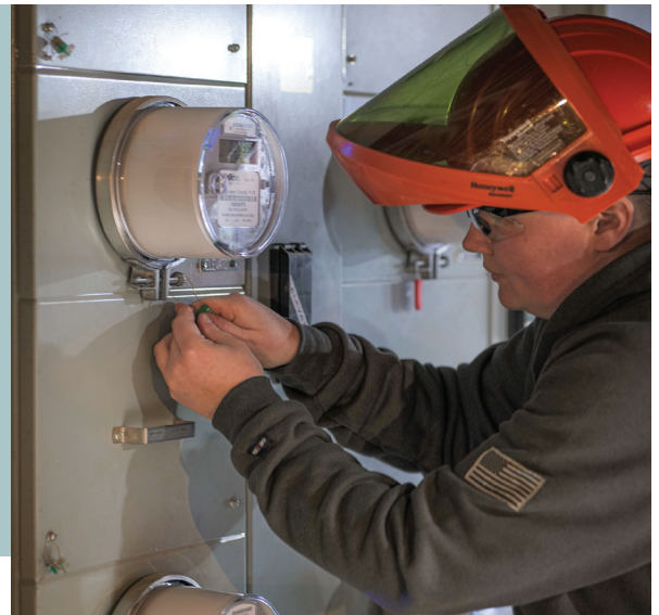
Metering Technician Corey Fletcher, attaches an anti-tamper tag to a new Vision meter. The meter pictured is part of a meter bank—a group of meters clustered together to serve separate units in a multi-tenant building.
