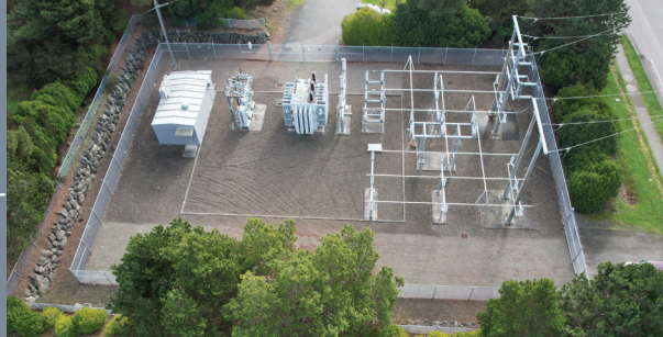
Infrastructure takes centerstage as our substations are upgraded to meet demand.
