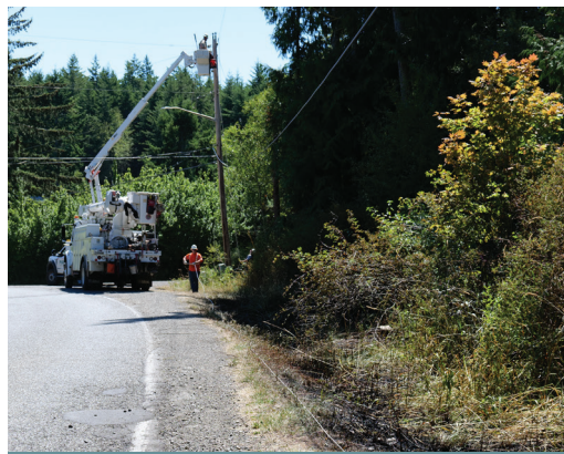
Line crew run new wire after a hazard tree beyond the utility right-of-way severed a line, igniting a brush fire.
